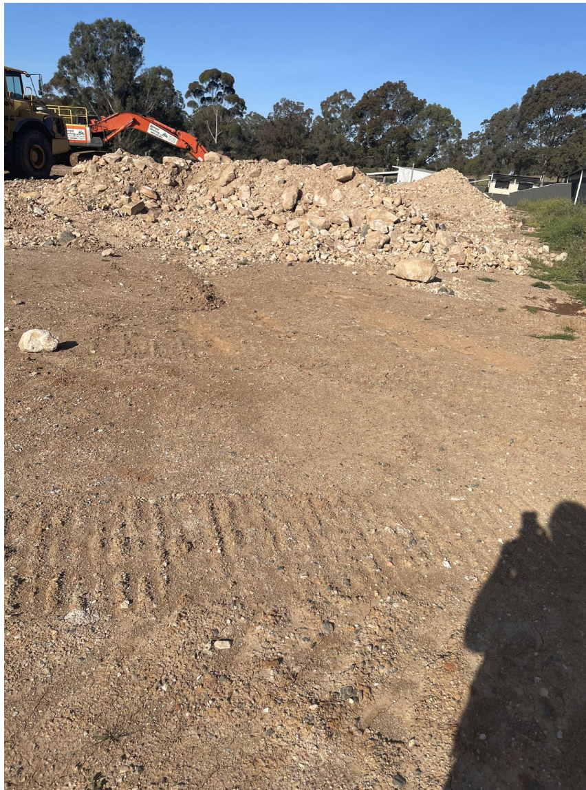
Photograph 6: Stockpile of Crushed Sandstone
